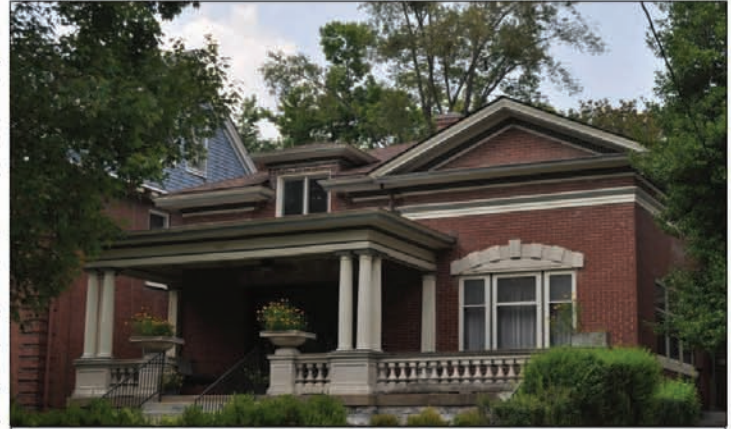
GARNER HOME BUILT BY HILLERICH FAMILY. (PHOTO BY JOHN ELGIN)
